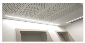
Assembly of the led strip HS14 in the recessed aluminum profiles for plasterboard with opal polycarbonate, this application makes the room illuminated in an excellent and stylish way.
