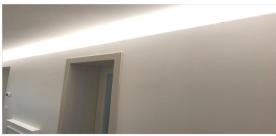
One architectural applications of the HS14 LED strip is to fix it inside of aluminum profile with opal polycarbonate cover, then mounted it facing upwards on a niche obtained in the plasterboard wall. The light is reflected from the ceiling and distributed effectively and without glare throughout the room.
